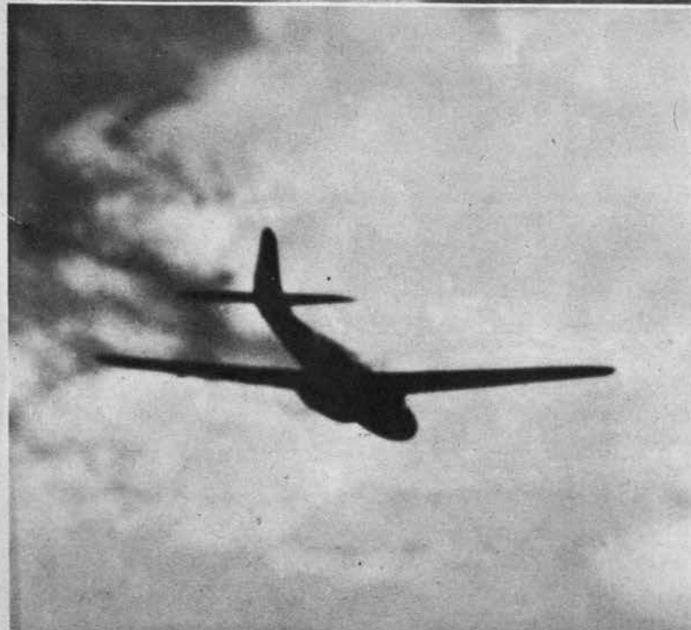
Action views from training film show the P-59A in various flying attitudes. Notable recognition features are its long broad wing, slender profile, upswept tail, and two close-set power units. No actual per-
